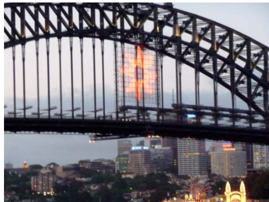
Sydney Harbour Bridge
