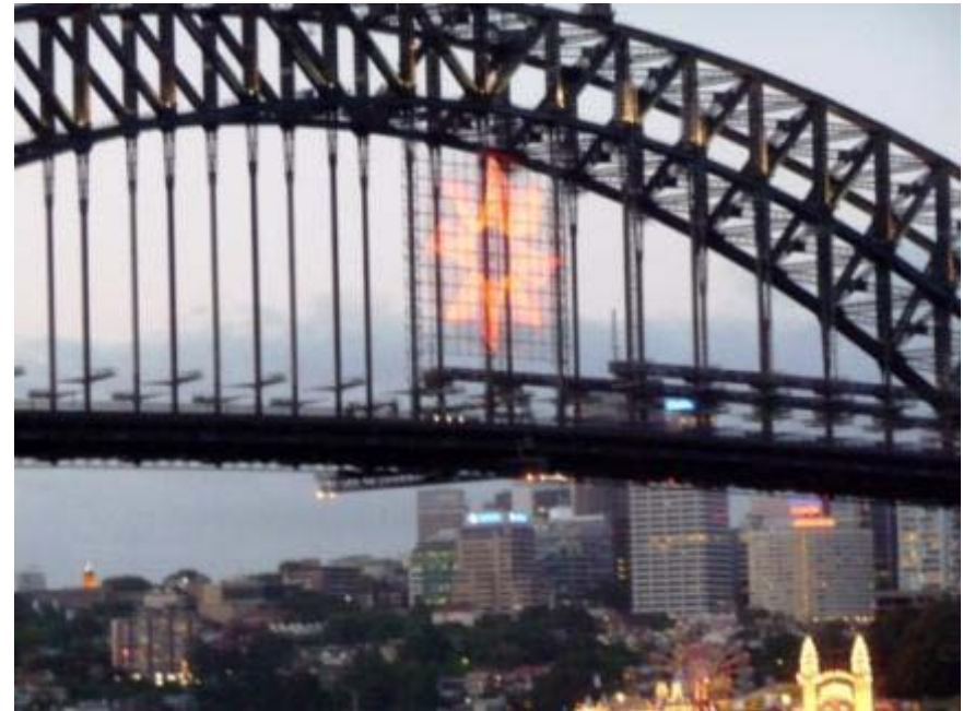
Sydney Harbour Bridge
